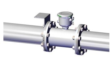
**Step 3:** Install mounting bracket, as positioned in the diagram, using the same meter installation bolts removed in Step 2.
