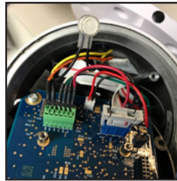
Splice black wires
