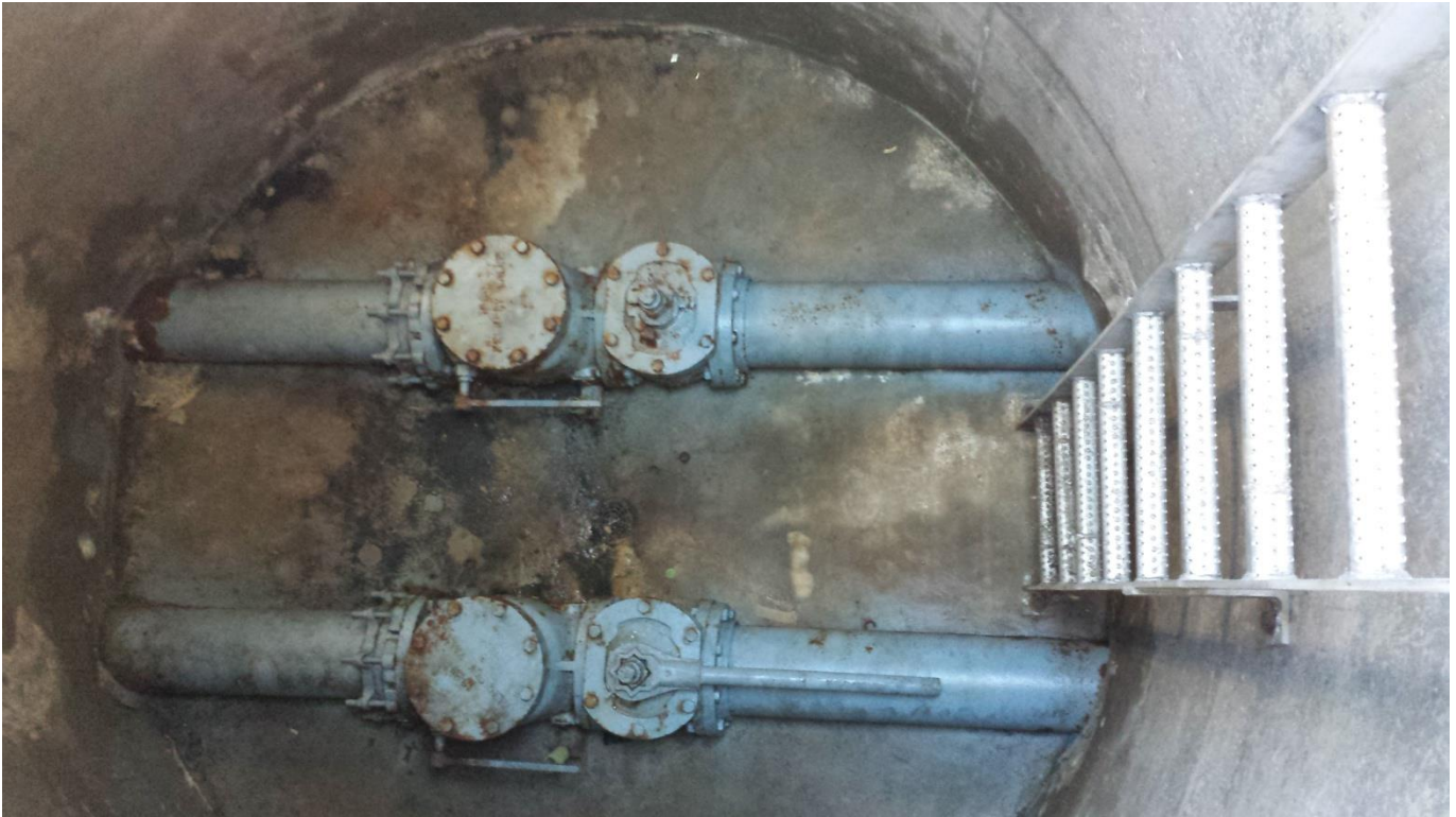
Figure 7 - Valve vault piping BEFORE installation
