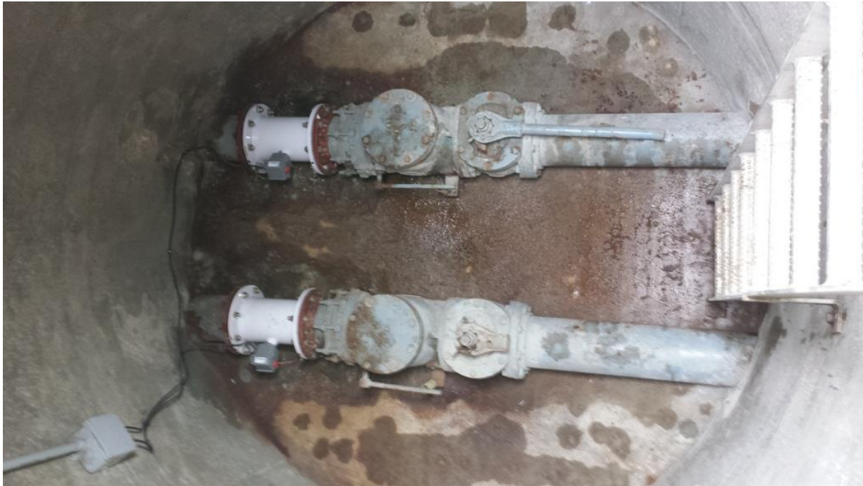
Figure 10 - Meters Installed
