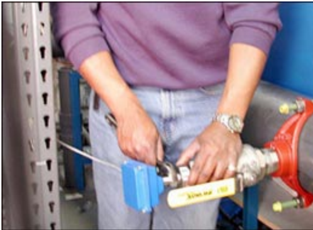
1. Loosen compression fitting
