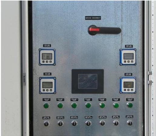
The FT420W Flow Computer processes the digital information, and resends the raw pulse output and an analog equivalent via 04-20ma loop outputs to the SCADA system, offering a smooth level of control for each VFD pump. In addition, the Flow Computer supplies a localized Flow Rate and Accumulated Total output for the site operator during inspection or troubleshooting. The distributed water is then filtered at each vineyard site and delivered to the vines via drip irrigation.
