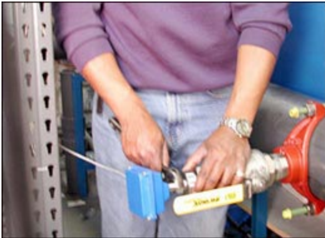
1. Loosen compression fitting
